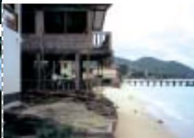
(top) This newly constructed building at Carriacou is on the beach and is very vulnerable to hurricane waves, 2000
