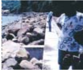
Hard engineering structures, such as this rock revetment at Victoria, Grenada, serve to protect the land, in this case, the coastal highway from erosion; but they do not promote the build-up of sand, 1999
